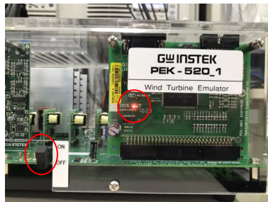
Figure 5.6 DSP normal status with light on
