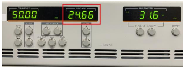
Figure 8.19 APS-300 voltage is bucked down to 24.66V
