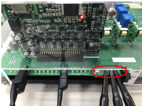
Figure 5.7 Oscilloscope test leads wiring
