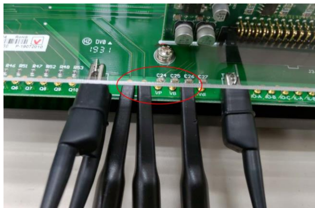
Figure 3.8 Oscilloscope test leads wiring
